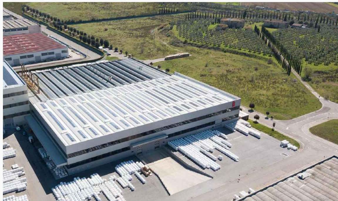
Aerial photo of the Sovigliana plant
